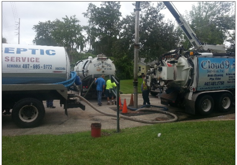
Figure 3. Vacuum Trucks in Service
